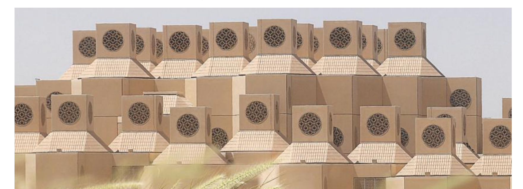
Modern Wind Towers at the Qatar University in Doha © Qatar University 14
